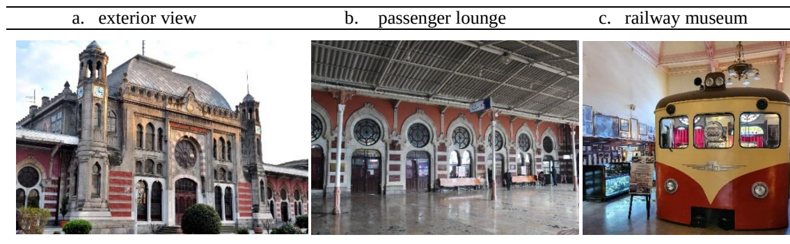
Figure 1. Partially decommissioned Sirkeci Train Station [(a): (Waldek, 2018)] [(b) and (c): (photo credit Ilke Ciritci, 2021)]
