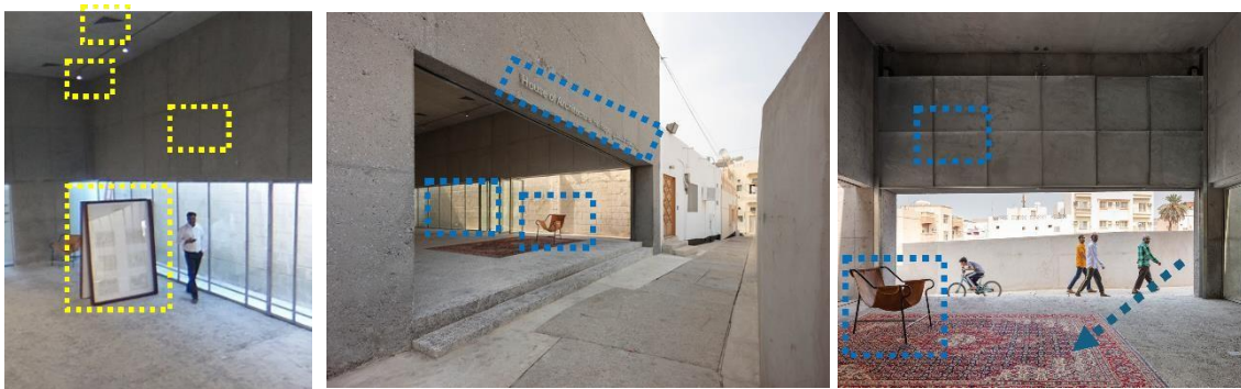
Figure 20. The concrete spans the entire plot width
