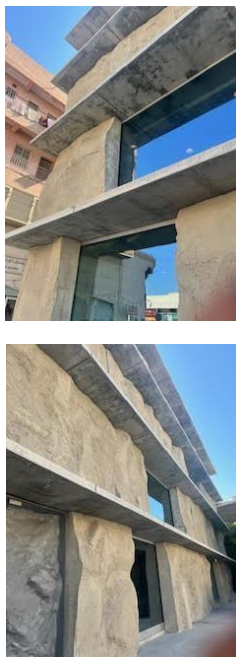
Figure 2. External image for the Green Corner building
