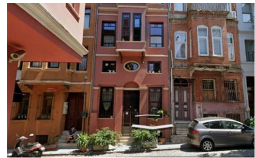
Figure 3. Building entrances with steps to the street Source: Öktem Karagül (2024)
