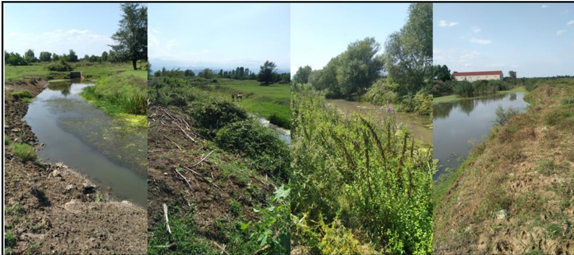
Figure 8. Processes of erosion and settlement of the soil massif of the collector slope
