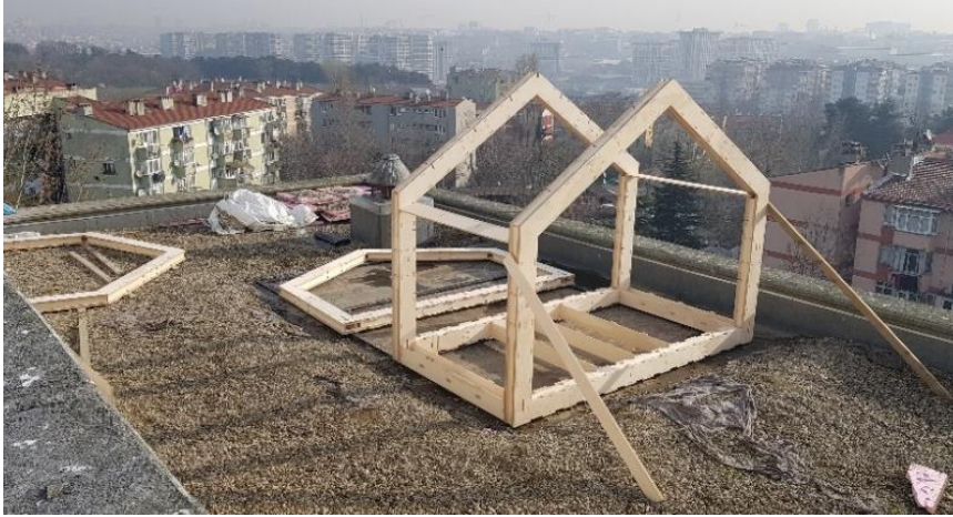
Figure 8. Assembly of the pentagonal supports and the floor connection components
